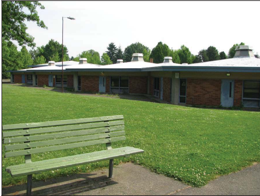
Figure 19: West elevation of the Clarendon School showing the school’s distinctive hexagonal “pod” unit design.
