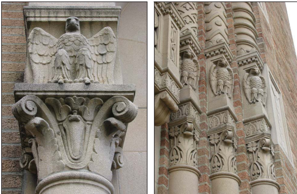
Figure 13. Cast stone detailing found near entryways at the Irvington School, 2009.
